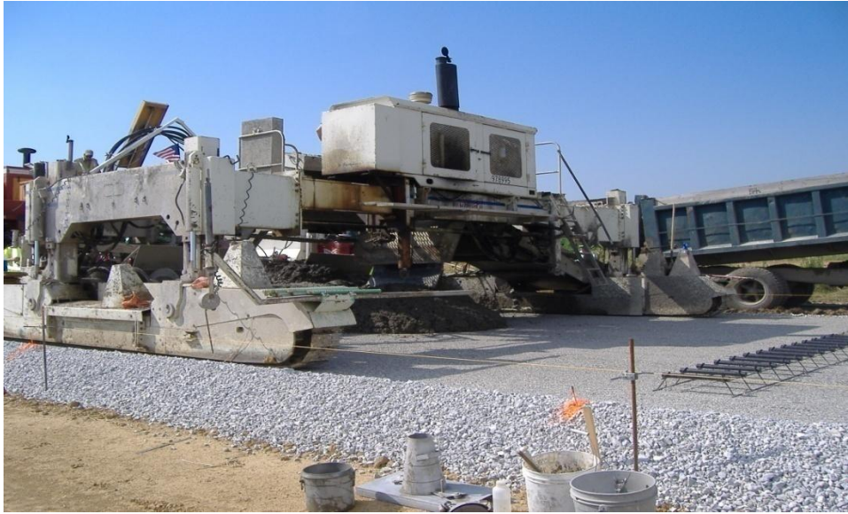
Figure 4.13 New Pavement Construction
